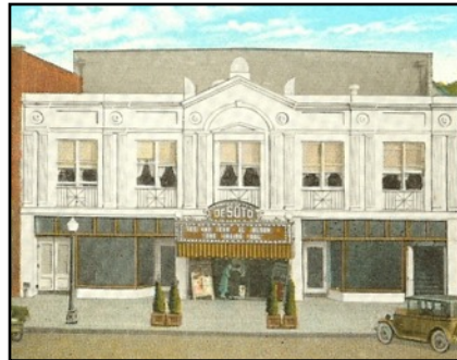
DeSoto 1929 Façade: The Historic DeSoto Theatre will go back to its original colors, as shown in the postcard from 1929.
