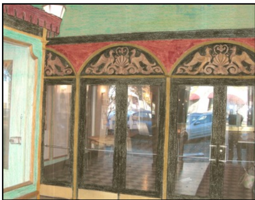
DeSoto Outside Entry: Outside entry picture colored over in the new colors. The facade project includes painting the Adam's style outside entry and the ticket kiosk back to their original colors. The doors will be high-gloss black, the trim and the griffins bright gold, the wall above the doors lacquer-red, and the walls green.
